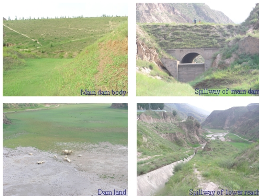
Figure 4.6. Major components of skeleton dam
